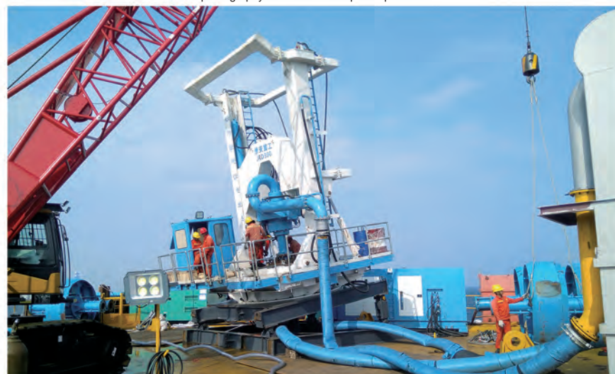
海上风电斜桩基础施工 Construction of inclined pile foundation for offshore wind power
