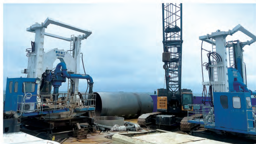
海上风电直桩基础施工 Construction of vertical pile foundation for offshore wind power
