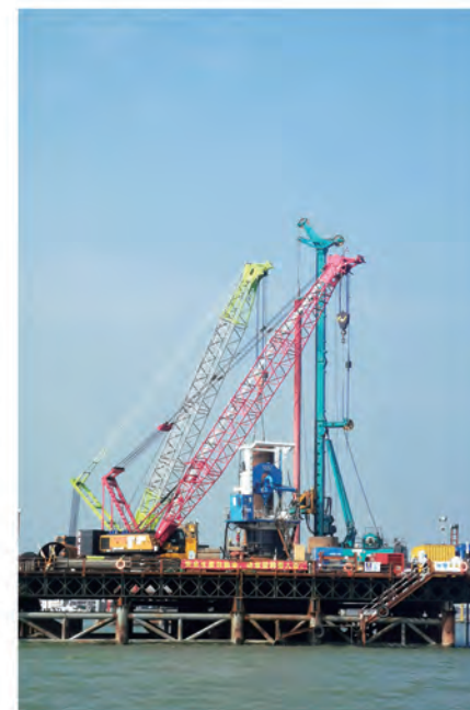
中国交建新加坡项目桩基施工 Offshore wind power pile foundation of China Jiaoqian in Singapore
