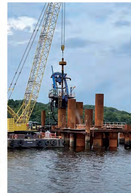
澳门四桥桩基施工 Offshore wind power pile foundation in Macau-Taipa Bridge
